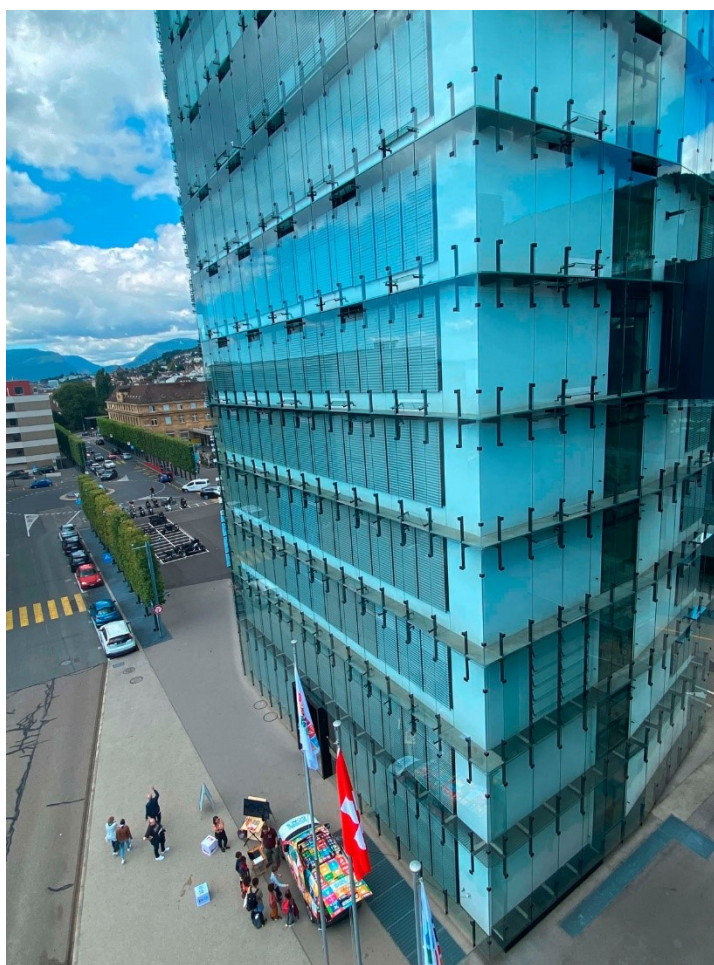
Picture 4: FSO building with SDG car at the FSO Open Day - picture taken by FSO
